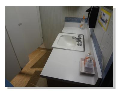
Photo -3 Most of the bathrooms have been updated to current accessibility standards, however this one inside the administration building is an example of the few that are in need of modernizing to meet accessibility standards
